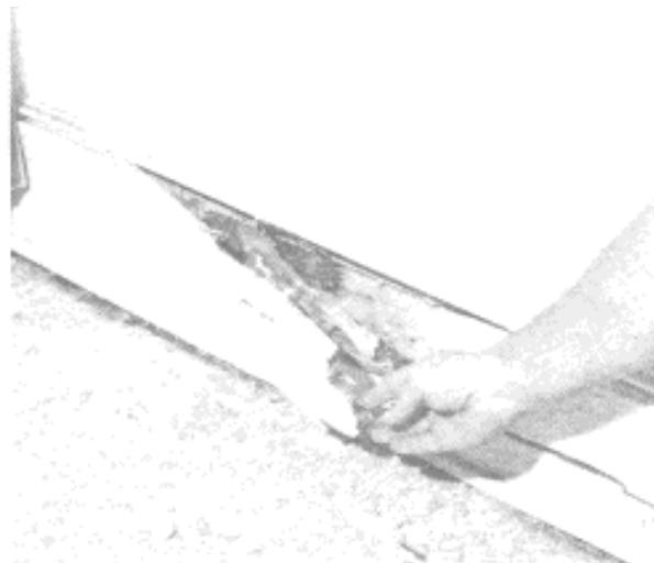
Figure 8. Decay in baseboard, often the first sign of Poria attack.
